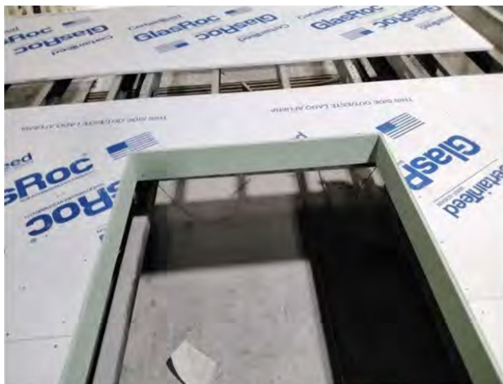
TBM-3 Thermal Break in window RO to reduce “flanking” around window frame
