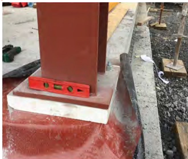
TBM-3 Thermal Break under support column
